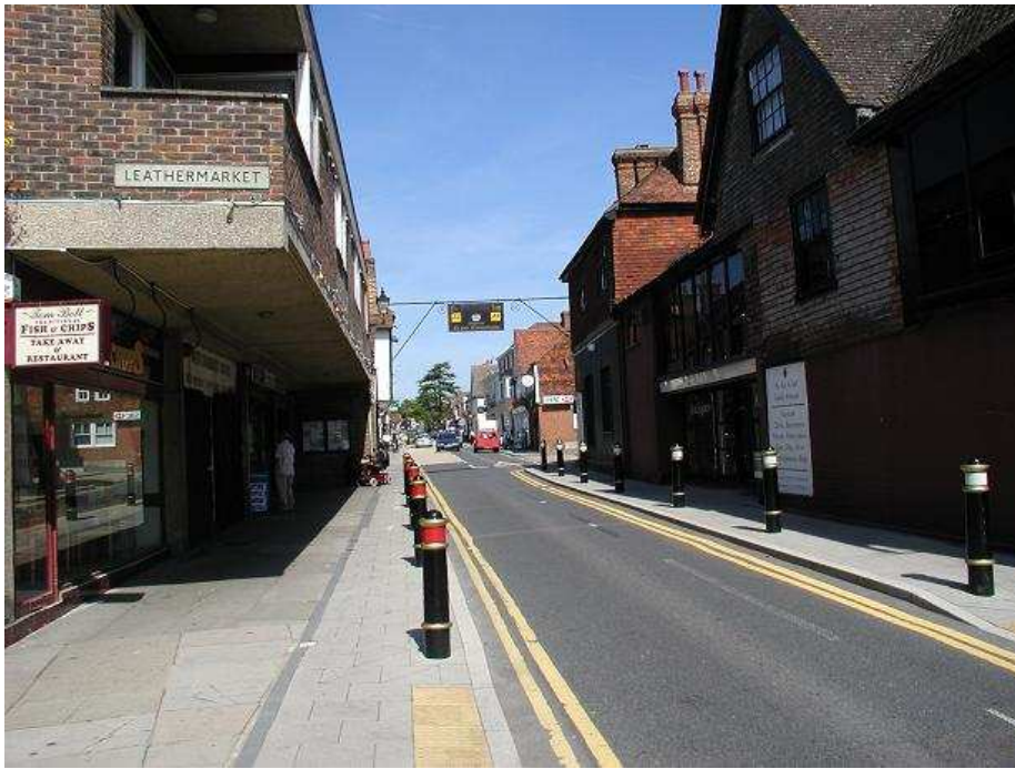
58 .prominent and distracting yellow lines
