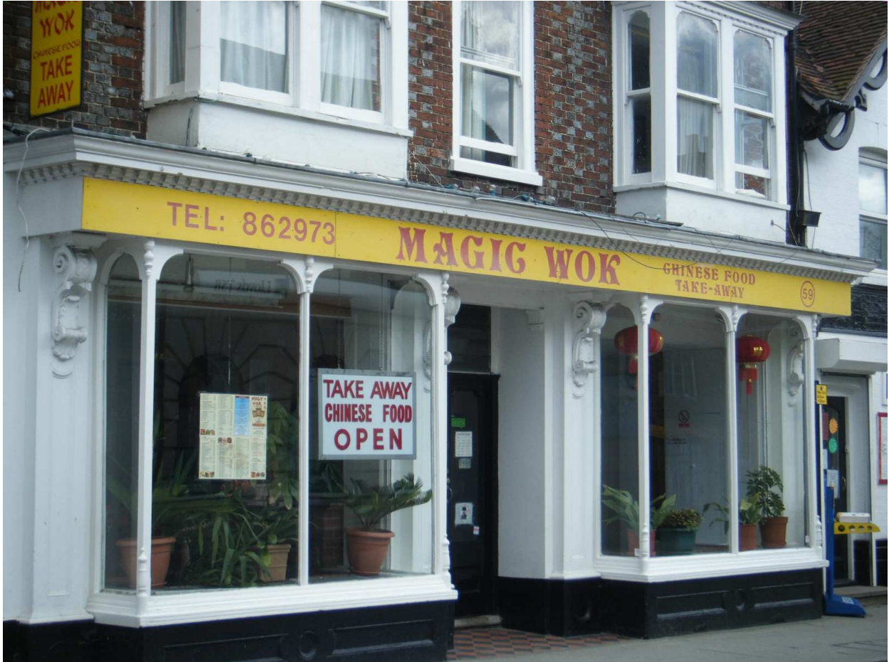
49. Another attractive shopfront in the High Street
