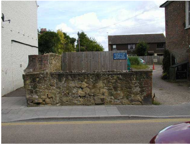
41. Portion of historic wall adjacent to No. 47
