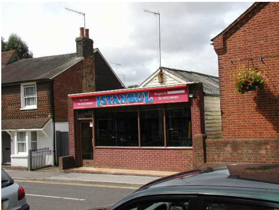
39 Unfortunate shopfront adjoining listed building
