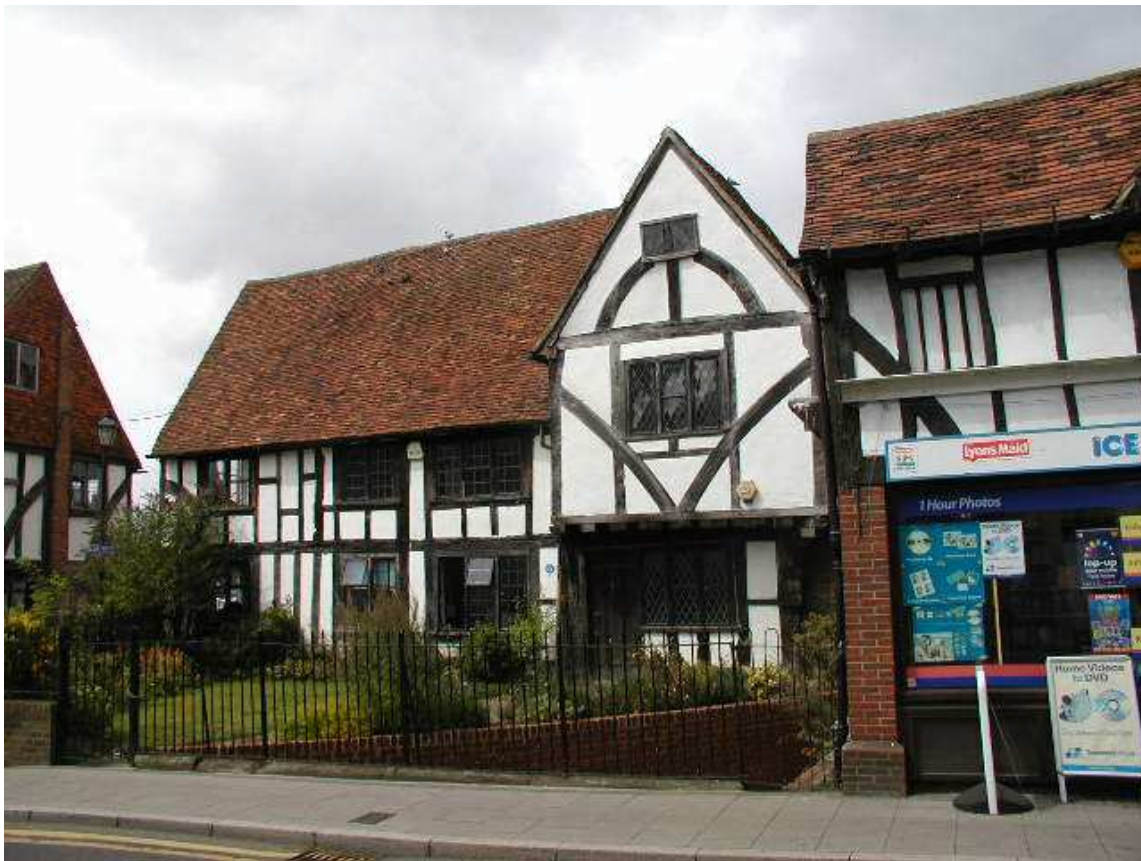
28. Typical Timber Framing to nos. 92 -94 High Street
