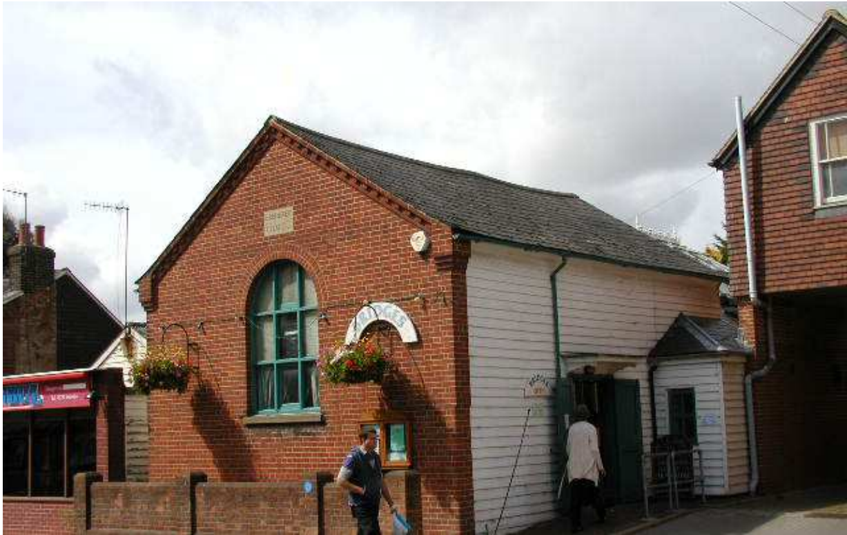
2. Historic ~Listed Chapel - now a community centre
